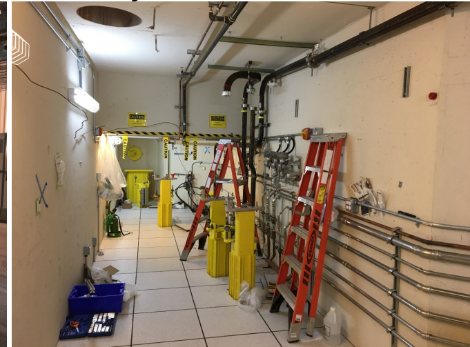
Gallery: Electrical circuits for new racks - done Magnet power supplies ready for cables
