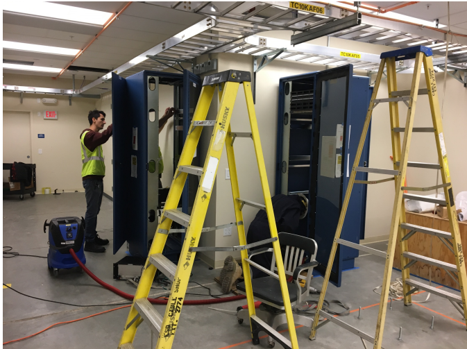
Laser Room: rack anchoring and laser controls installation
