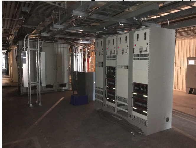
Gallery: Electrical circuits for new racks - done Magnet power supplies ready for cables
